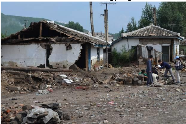
Photo 3: Devastation of household by the flood in Hoeryong.
