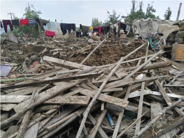
Photo 13: Devastation of household by the flood in Hoeryong.
