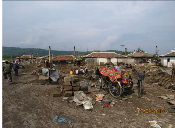
Photo 8: Devastation of household by the flood in Hoeryong.
