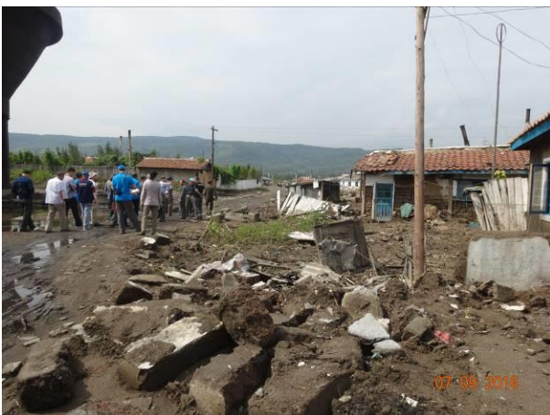
Photo 5: Devastation of household by the flood in Hoeryong.
