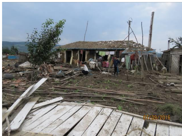
Photo 10: Devastation of household by the flood in Hoeryong.
